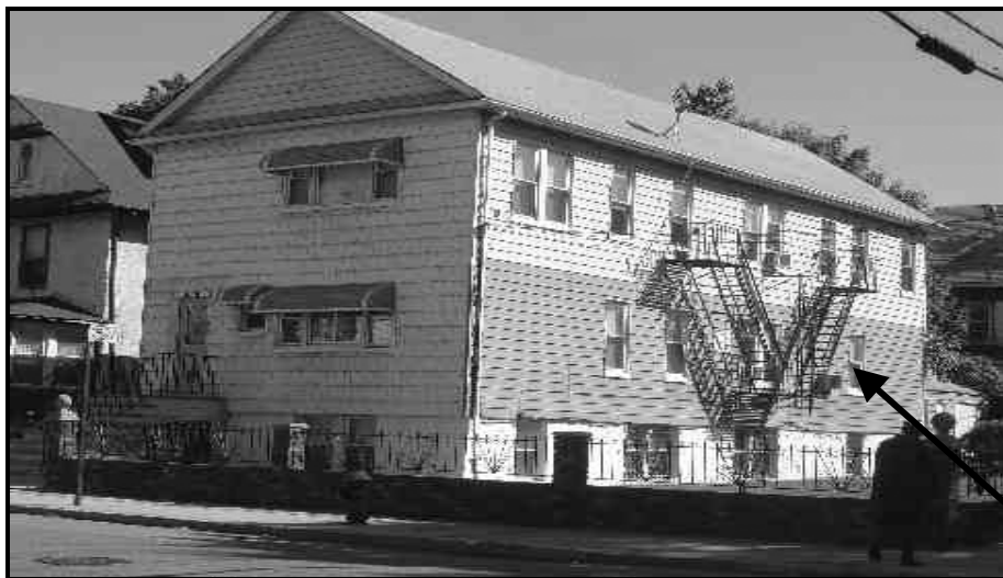
Figure 5. The fire escapes suggest several housing units. There are also signs of basement apartments.
