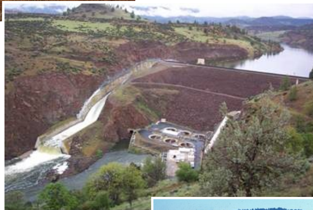
Iron Gate Dam on the Klamath River
