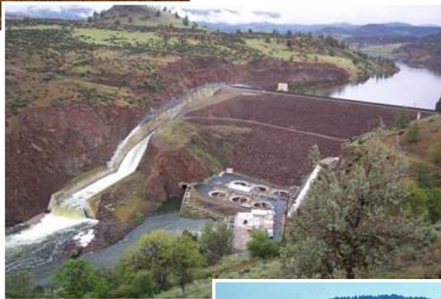
Iron Gate Dam on the Klamath River
