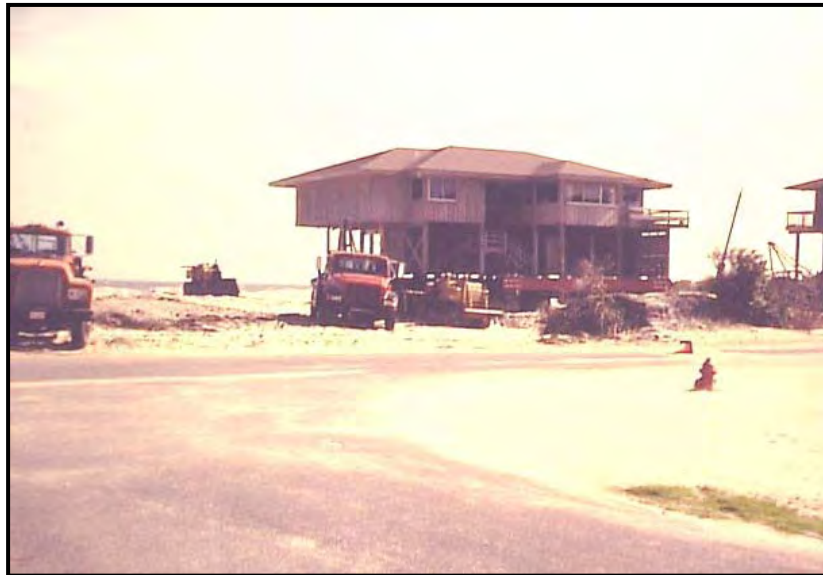
Building being relocated from the erosion hazard area after Hurricane Fran, Figure Eight Island, North Carolina (photo from Berry Williams).
