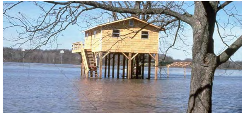
This house was elevated and the lower area was not enclosed. There was no flood damage to the structure.
