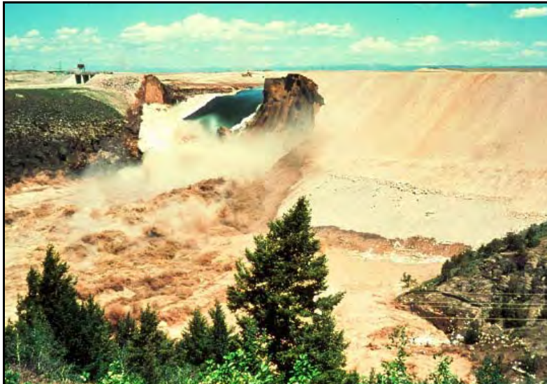
View northwest toward the breach in Teton Dam (Idaho) during the dam's failure. The canyon floor is flooded from bank to bank, and all works there are completely inundated. Photo by Mrs. Eunice Olson (Sylvester, 2006).
