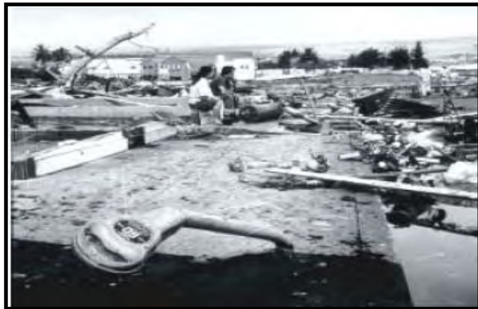
Damage from the 1960 tsunami in the Waiakea area of Hilo, Hawaii. The force of the debris-filled waves bent parking meters. (National Tsunami Hazard Mitigation Program, 2001, p. 13; Photo from U.S. Navy.)
