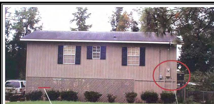
Flood protection elevation
