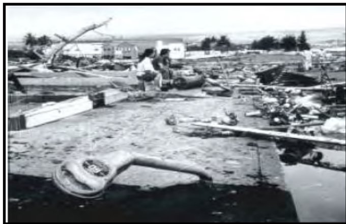
Damage from the 1960 tsunami in the Waiakea area of Hilo, Hawaii. The force of the debris-filled waves bent parking meters. (National Tsunami Hazard Mitigation Program, 2001, p. 13; Photo from U.S. Navy.)
