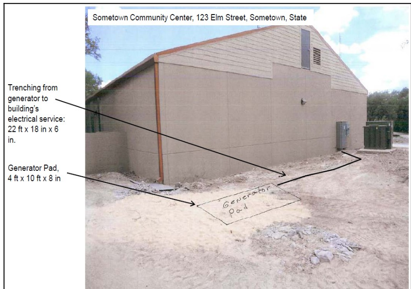
Figure 4. Ground-level photograph showing proposed ground disturbance area.
