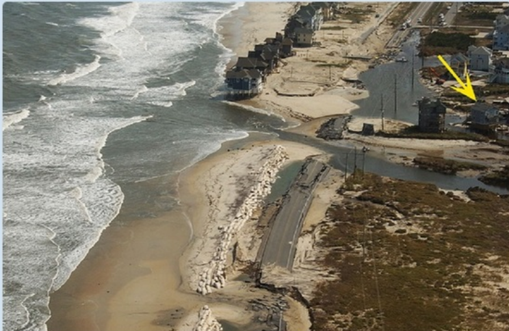
Rodanthe, NC. Hurricane Sandy caused this section of coastline to experience inundation with resulting damage to housing and infrastructure.
