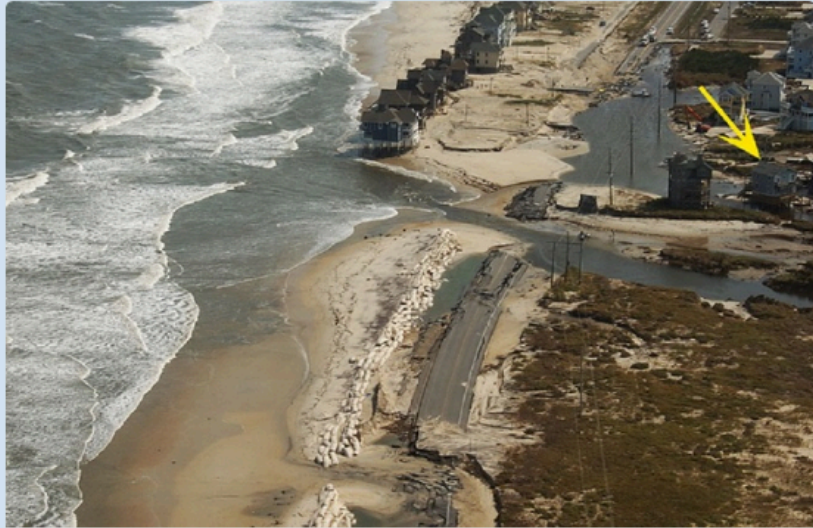
Rodanthe, NC. Hurricane Sandy caused this section of coastline to experience inundation with resulting damage to housing and infrastructure.
