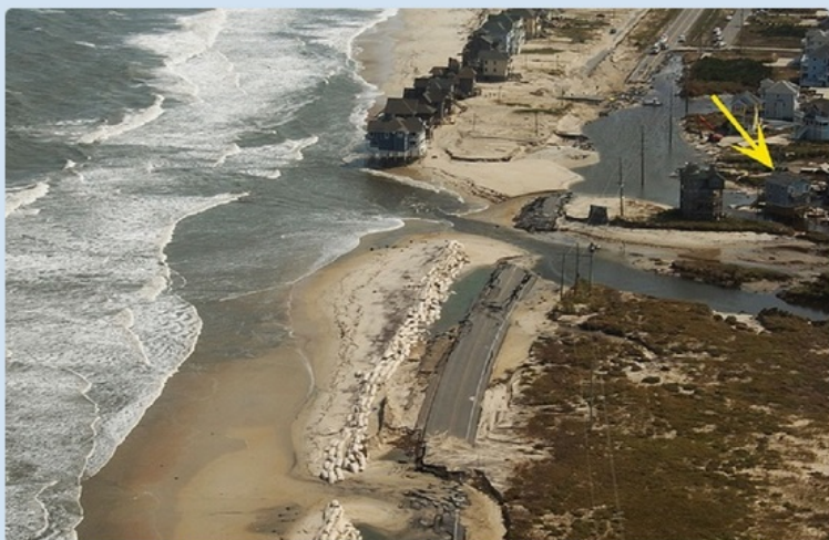
Rodanthe, NC. Hurricane Sandy caused this section of coastline to experience inundation with resulting damage to housing and infrastructure.
