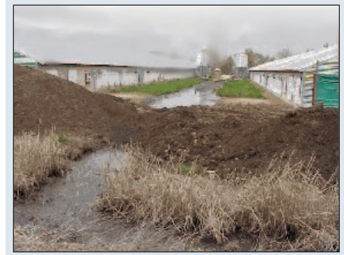
Storage facility maintenance is essential. (Source: EPA Region 10)
