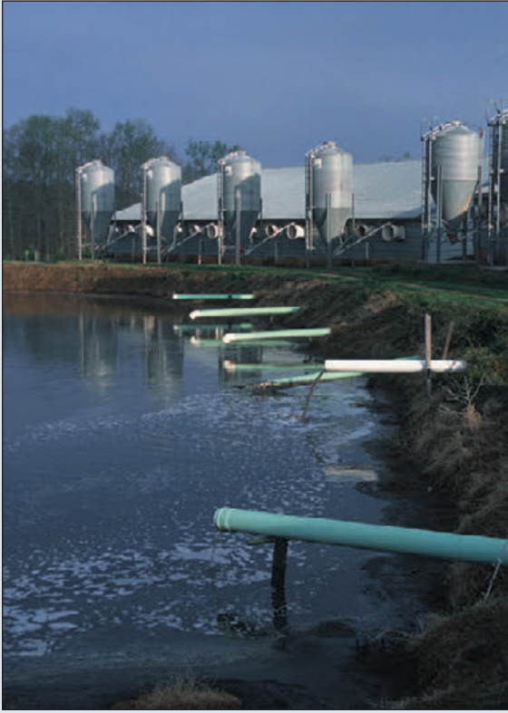
An automated lagoon waste management system for a 900-head hog farm. (Photo courtesy of USDA/NRCS)
