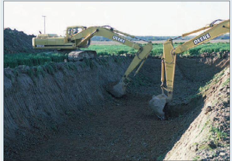
Construction of a storage pond at a farm in Lonoke County, Arkansas. (Photo courtesy of USDA/NRCS)
