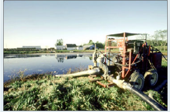
CAFO waste lagoon—a liquid manure storage structure. (Photo courtesy of USDA/MO NRCS)
