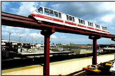
Monorail/Automated Guideway (MG) Rail – Fixed Guideway
