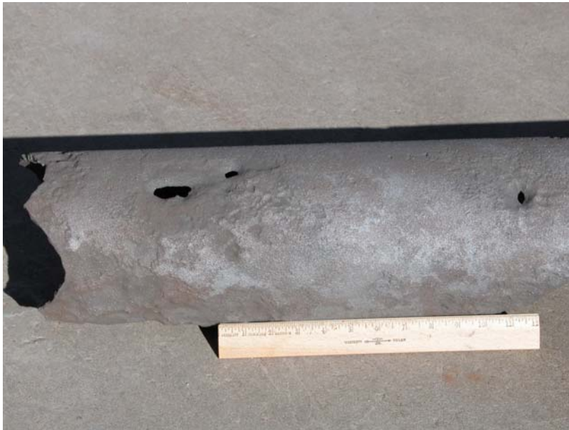
Figure 2: Same pipe section as shown in Figure 1 after sand blasting. Note extensive metal loss and the perforation of the pipe wall at three locations. This example demonstrates the difficulty in visually identifying areas which that have experienced graphitic corrosion.
