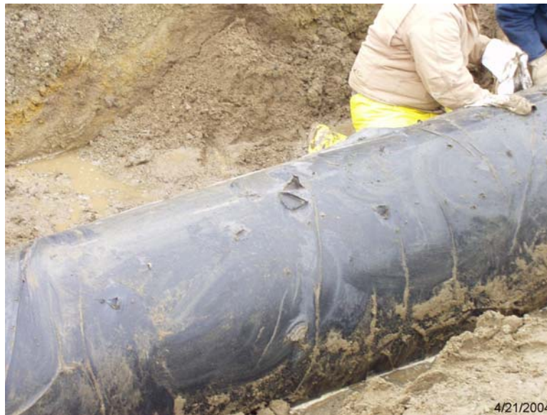
Figure 1—Excavated 30-inch diameter Southwest pipe unit with PE encasement
