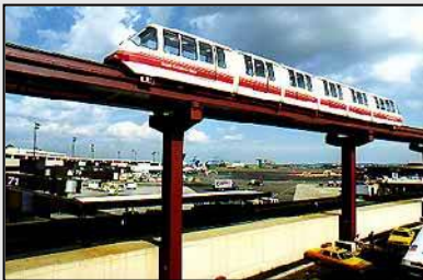
Monorail/Automated Guideway (MG) Rail – Fixed Guideway
