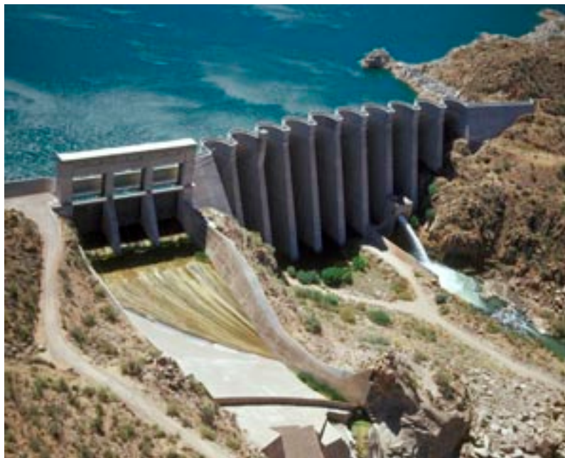
Figure 6. Concrete Multi-Arch Dam (Bartlett Dam. U.S. Bureau of Reclamation; Photo: National Park Service, 2013)
