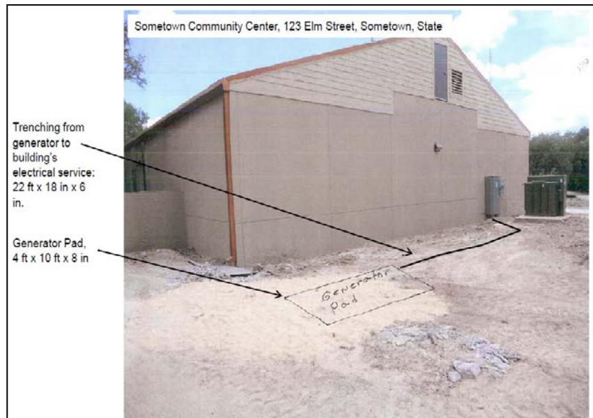
Figure 4. Ground-level photograph showing proposed ground disturbance area.
