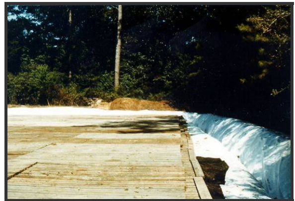
Shown above, the ring levee and wellpad are covered with a plastic liner and board mats are placed on the liner. Equipment is placed on primary liner (below).
