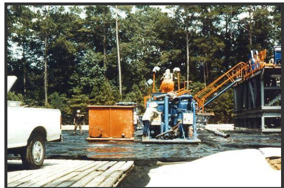
Shown above, the ring levee and wellpad are covered with a plastic liner and board mats are placed on the liner. Equipment is placed on primary liner (below).
