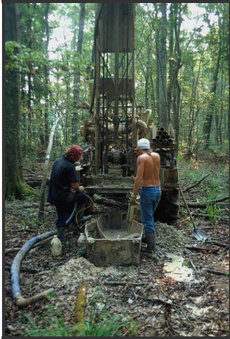
In this photo, trails were cut to provide access for large drilling equipment.
