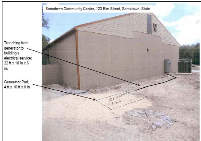
Figure 4. Ground-level photograph showing proposed ground disturbance area.
