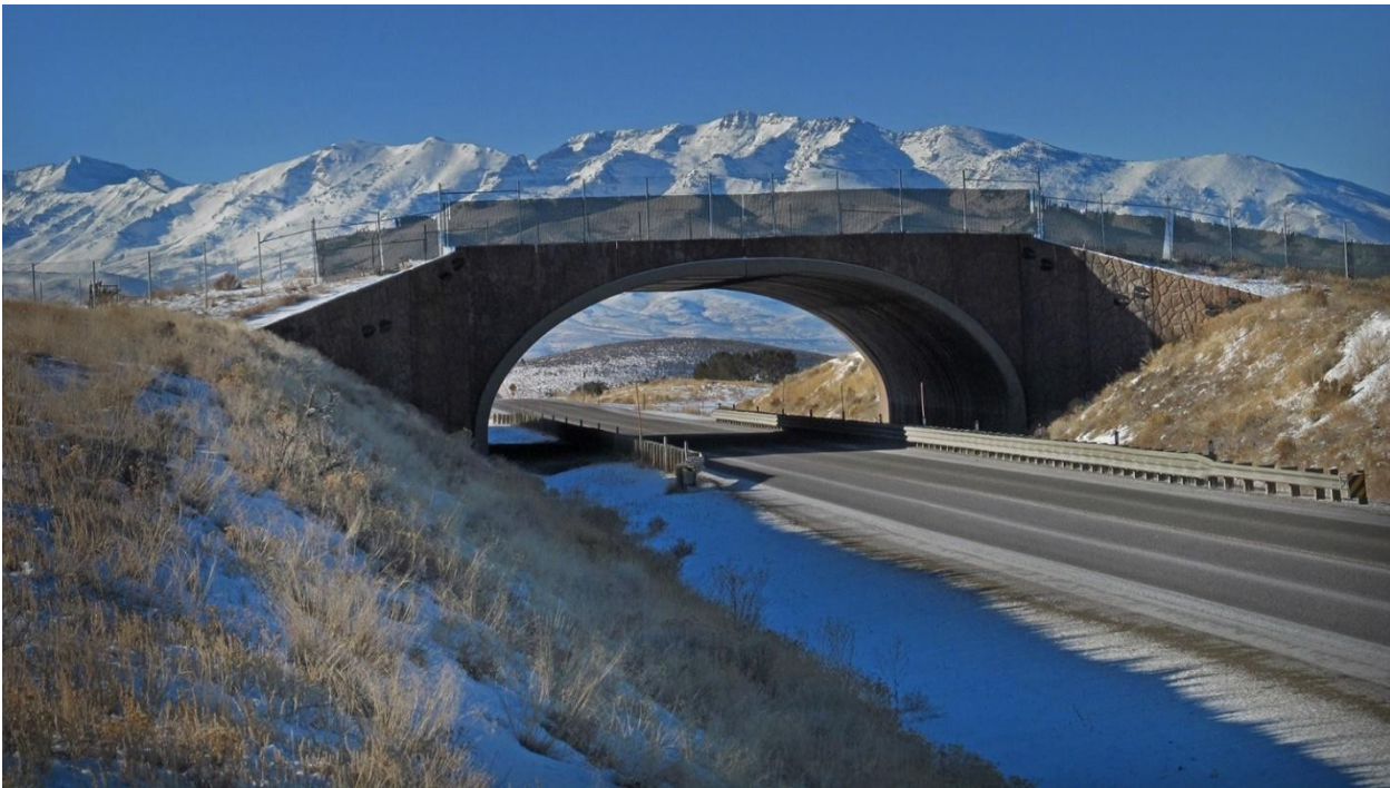
State and federal partners, through the Wildlife Sport Fish Restoration Program, have built and are now monitoring the effectiveness of the wildlife overpass project seen here along Highway 93, in Elko County, Nevada.
