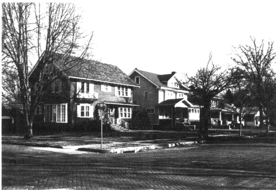
The Barnard Park Historic District, Fremont, Dodge County, Nebraska, contains 187 upper and middle class homes constructed between 1870 and 1929. It typifies the early development of residential neighborhoods in small towns on the Great Plains. (Joni Gilkerson).
