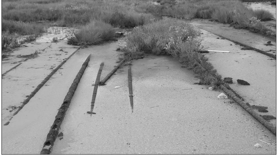
Figure 9: Examples of Unreclaimed Infrastructure on NWRs
