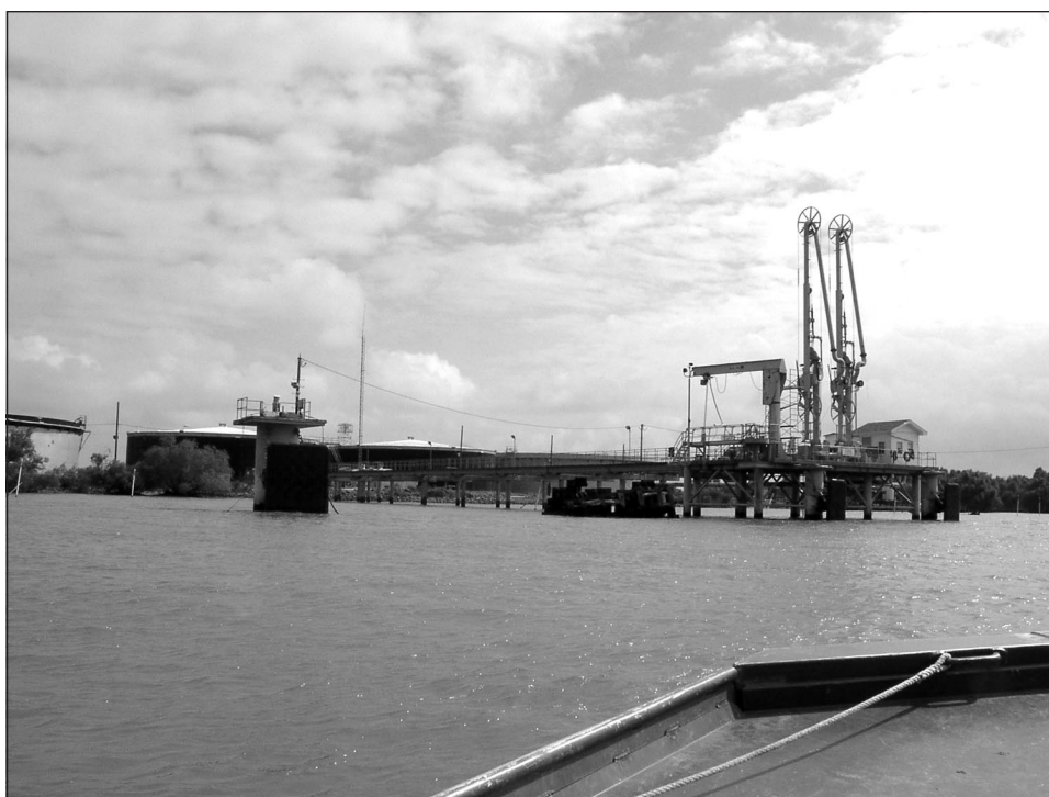
Figure 3: Pipeline Storage and Loading Facilities, Delta NWR (La.)
