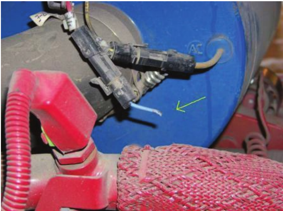
BROKEN "F1" WIRE IN THE ALTERNATOR (3,396 TEST MILES)
