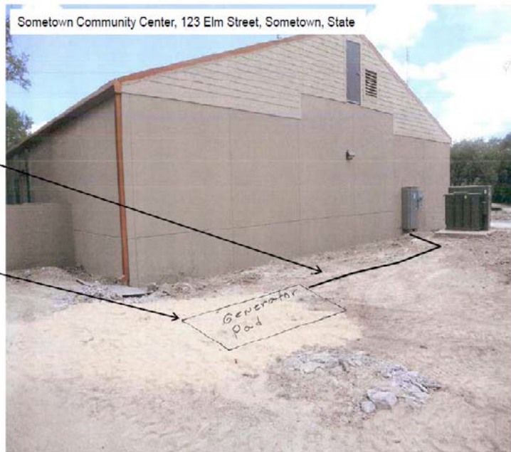
Figure 4. Ground-level photograph showing proposed ground disturbance area.
