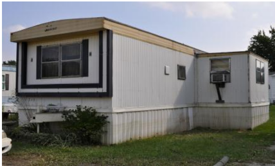
The visible water line is below the floor system.
