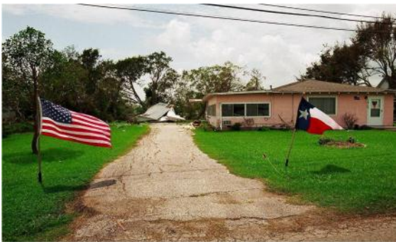
Only an outbuilding has sustained damage.
