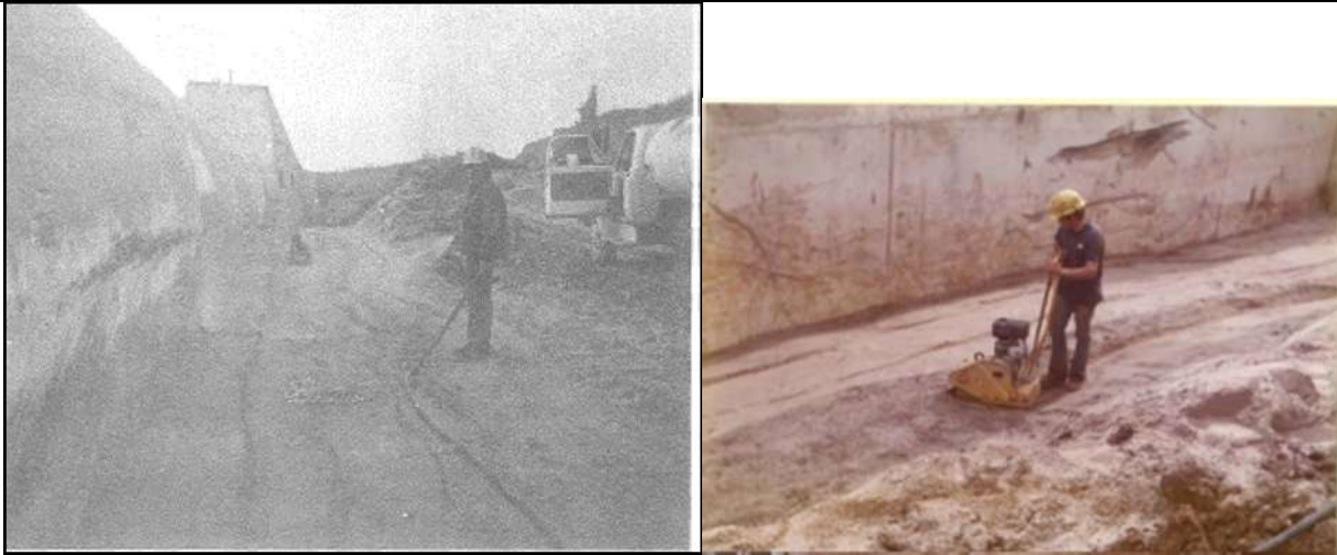
Construction Photographs of Filter Placement around the Conduit
