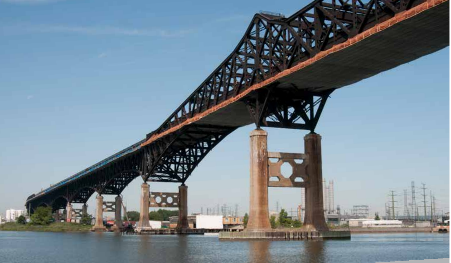
Pulaski Skyway between Jersey City, Hudson County and Newark, Essex County
