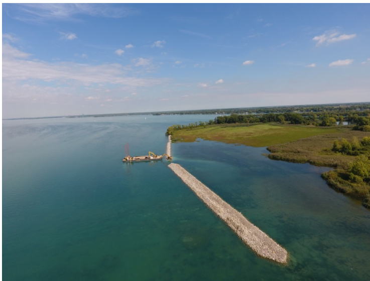
Figure 7. Stony Island north shoal restoration.
