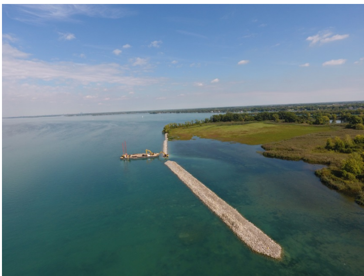
Figure 7. Stony Island north shoal restoration.
