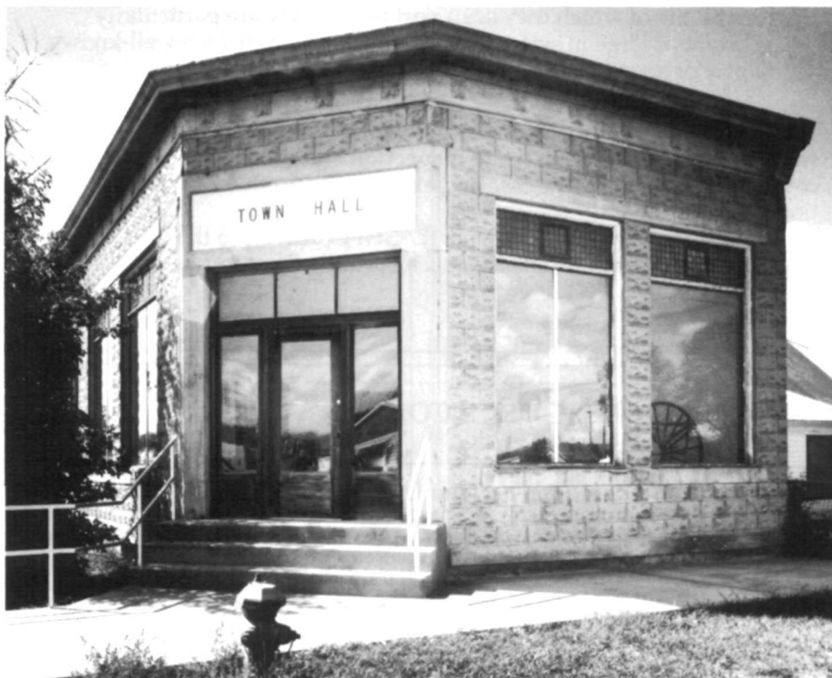
Functions and uses often change. Built as the Stockgrowers Bank in 1916, this building in Carbon County, Wyoming, became the Dixon Town Hall in 1975. By serving the region's farmers and ranchers from 1916 to 1923, the bank played an important role in fostering the frontier town's development. (Richard Collier)
