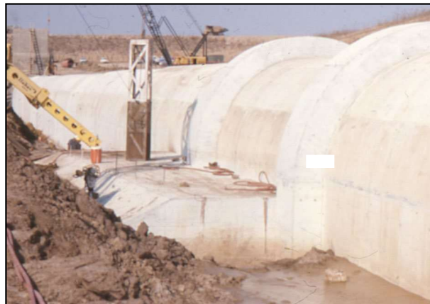
Portion of concrete plug along conduit
