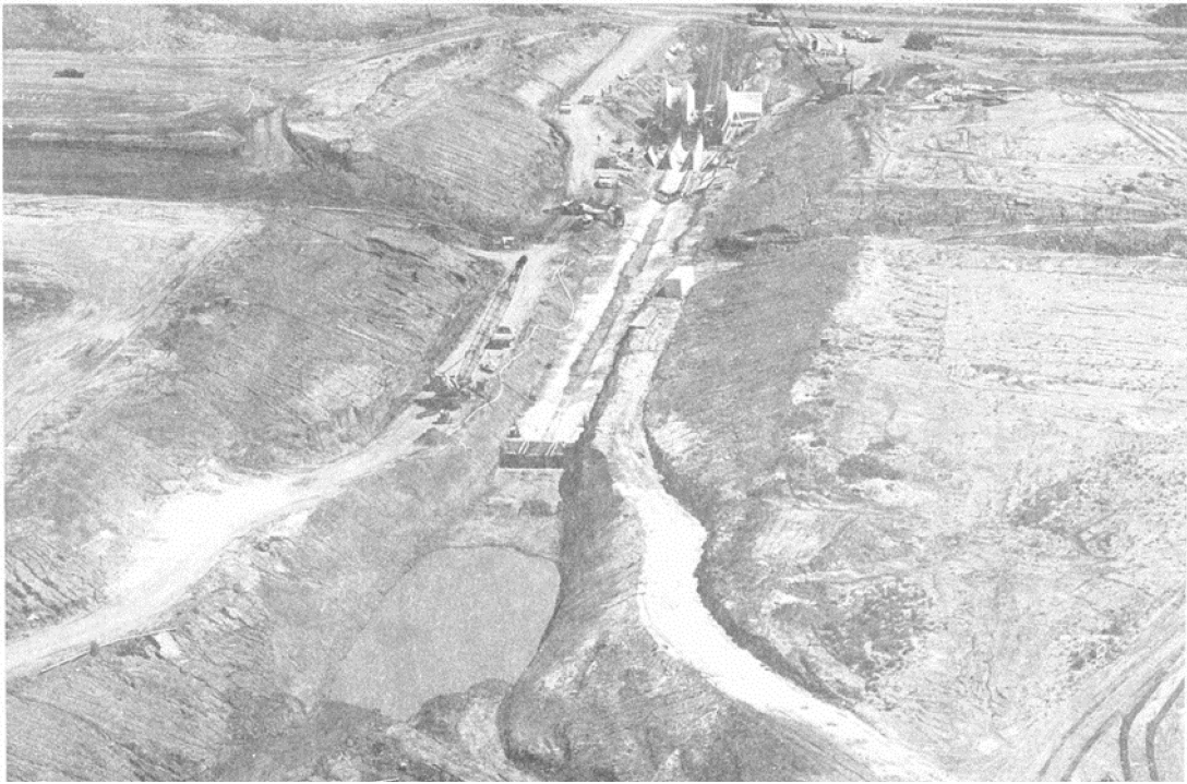
Construction Photograph of Outlet Works Excavation
