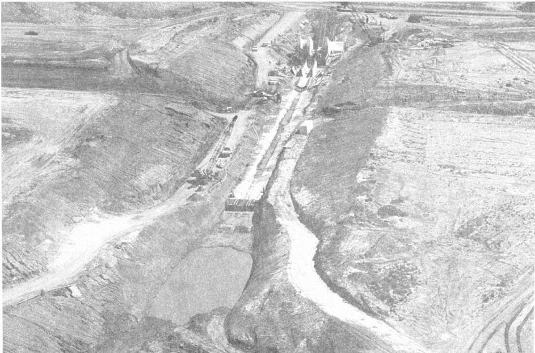
Construction Photograph of Outlet Works Excavation
