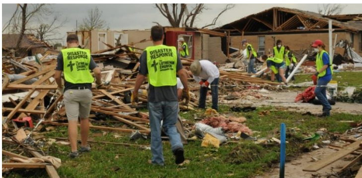
Moore, OK, May 26, 2013 – Volunteers with the Missouri Lutheran Church Disaster Response team help survivors clean up after a deadly tornado. Volunteers provided much needed personal services and were important FEMA partners in disaster recovery. Photo by George Armstrong/FEMA
