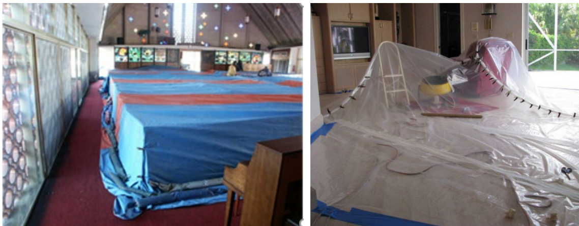
Fig. 5. Tarped pews in church fumigated for control of drywood termites (left, photo by Rudi Scheffrahn), tarped hardwood flooring fumigated for drywood termite control (right).
