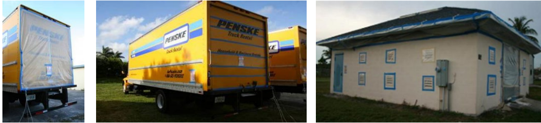
Fig. 7. Tape-and-seal (photos left to right); truck cargo containers (two methods of tape-and-sealing), concrete block garage.
