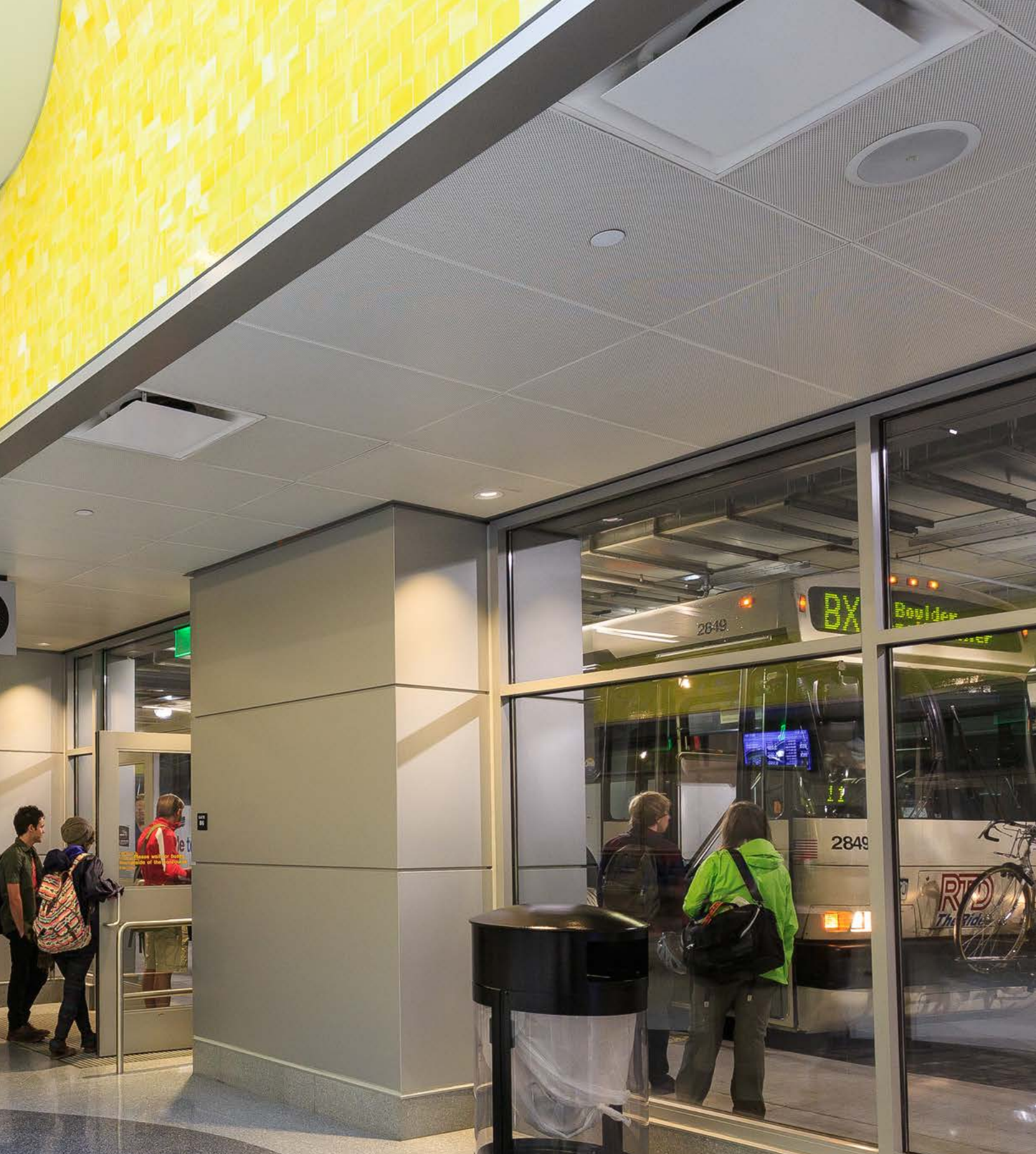
Part of the Union Station Transit Center, RTD's 22-gate underground bus facility provides convenient connections across the system. Photo credit: RTD.
