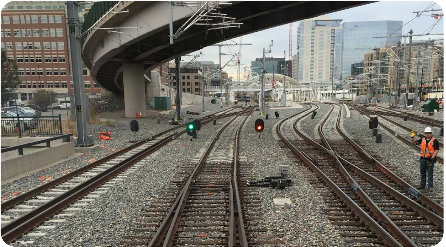
As a relatively young agency, RTD has not experienced the decaying infrastructure that many older and larger transit systems have. Photo credit: RTD.
