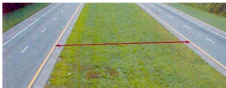
Figure 26: Median Width Measurement
