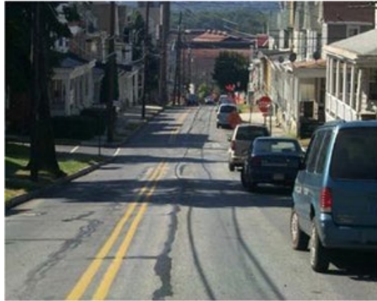
Figure 87: No Widening Potential (Code 1)
