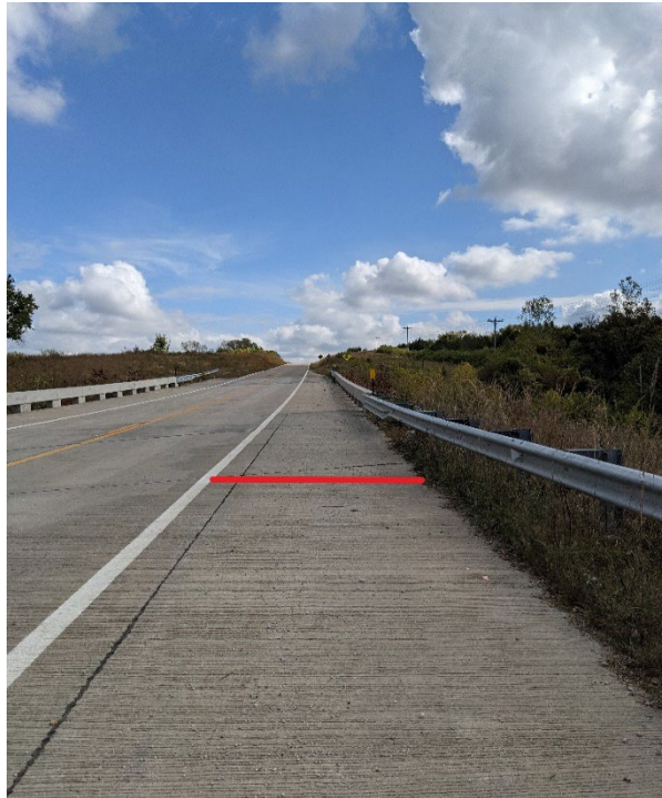
Figure 33: Measuring Shoulders with Guardrails
