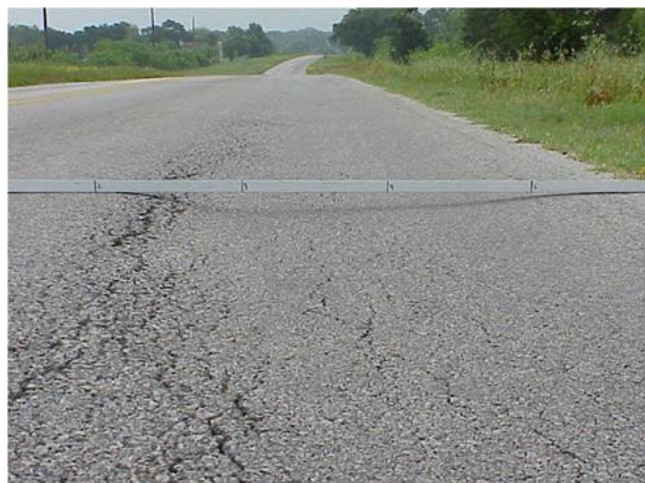
Figure 65: Rutting Example
