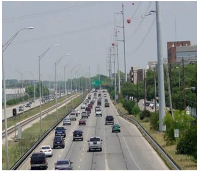
Figure 90: Major Rail Line (Code B) Obstacle Example
