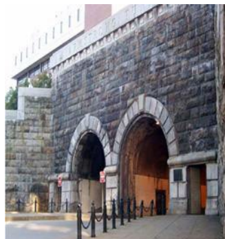
Figure 16: Tunnel (Code 2) Example
