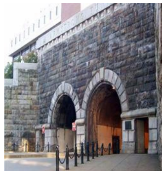
Figure 16: Tunnel (Code 2) Example
