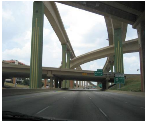
Figure 61: Full Access Control (Code 1) Examples All access via grade-separated interchanges
