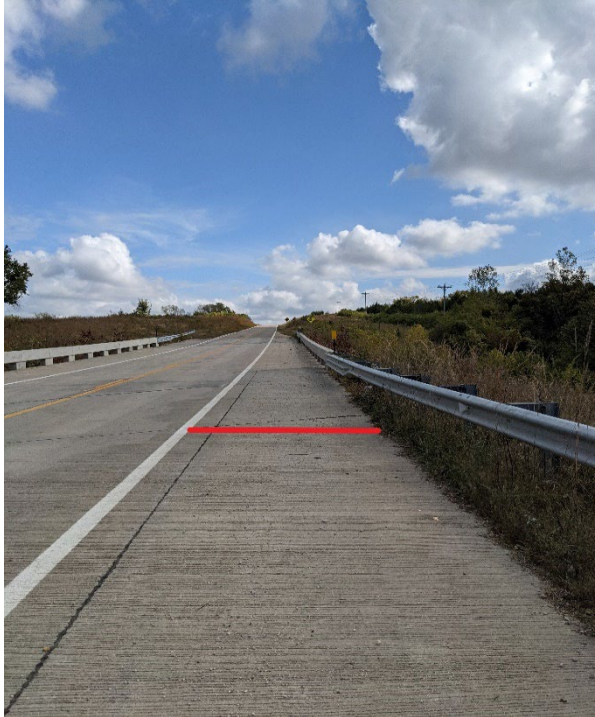
Figure 33: Measuring Shoulders with Guardrails
