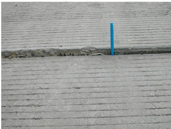
Figure 67: Faulting Example
