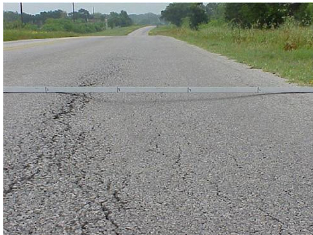
Figure 65: Rutting Example
