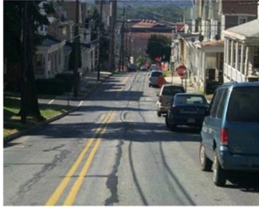
Figure 87: No Widening Potential (Code 1)
