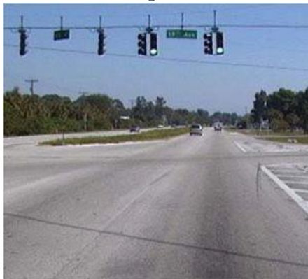
Figure 53: Uncoordinated Fixed Time (Code 1) Example
