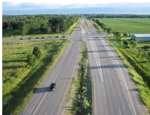
Figure 62: Partial Access Control (Code 2) Examples Access via grade-separated interchanges and direct access roadways
