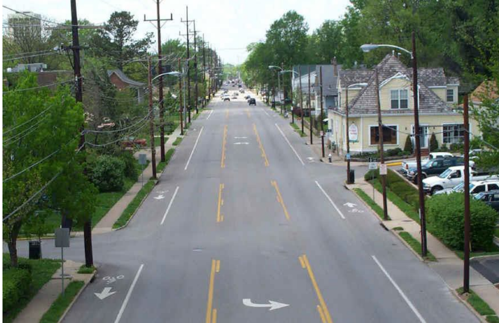
Source: Kentucky Transportation Cabinet
