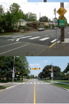
$\circ Mid\text{-}block$  crossings with <u>pedestrian hybrid beacons</u> or <u>rapid rectangular flashing beacons</u>
