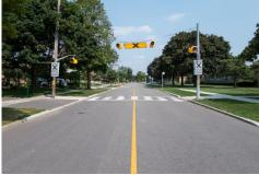
OMid-block crossings without pedestrian hybrid beacons or rapid rectangular flashing beacons
