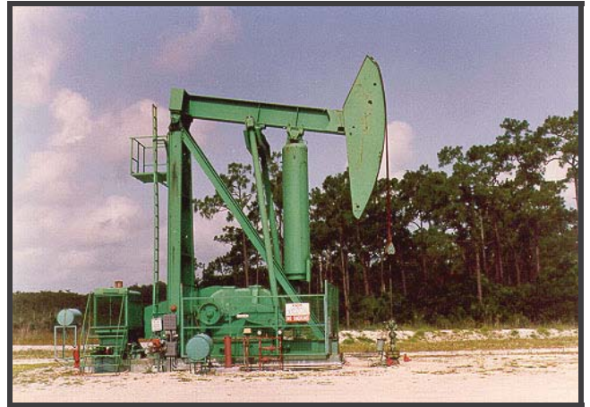
A well-maintained pump jack operation...
