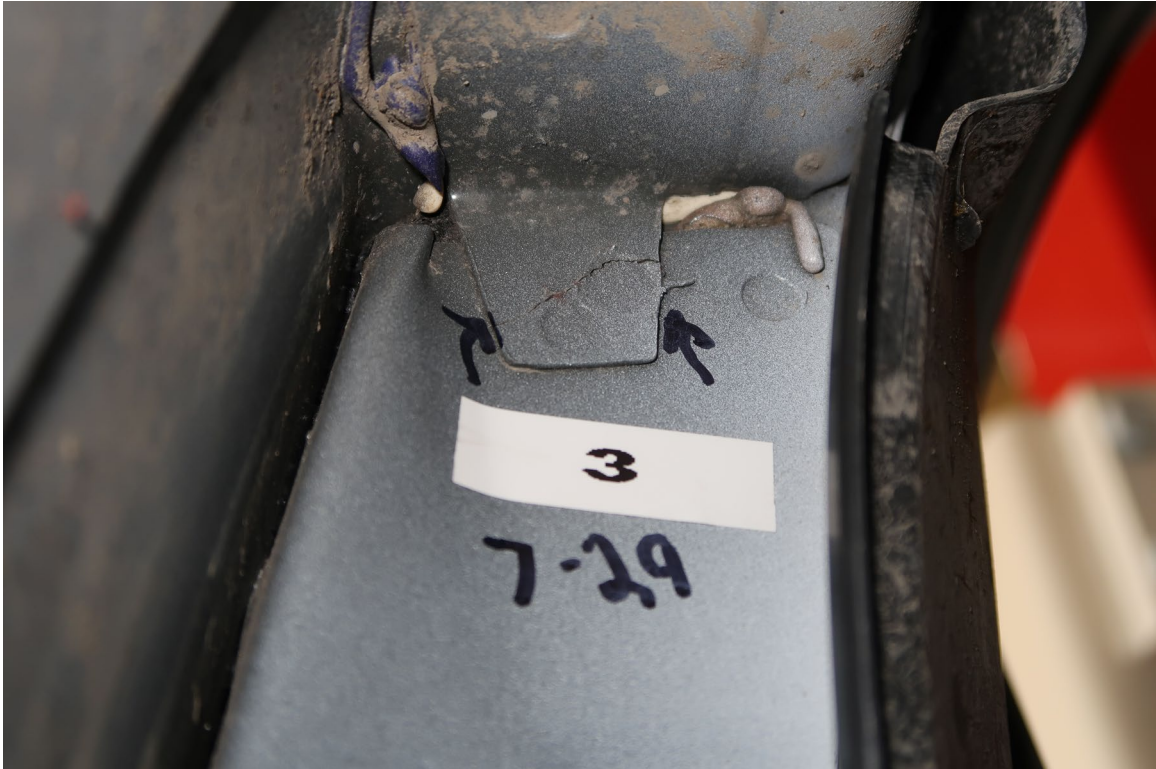
CRACK #3; CRACK IN THE BODY UNDER THE STEP
