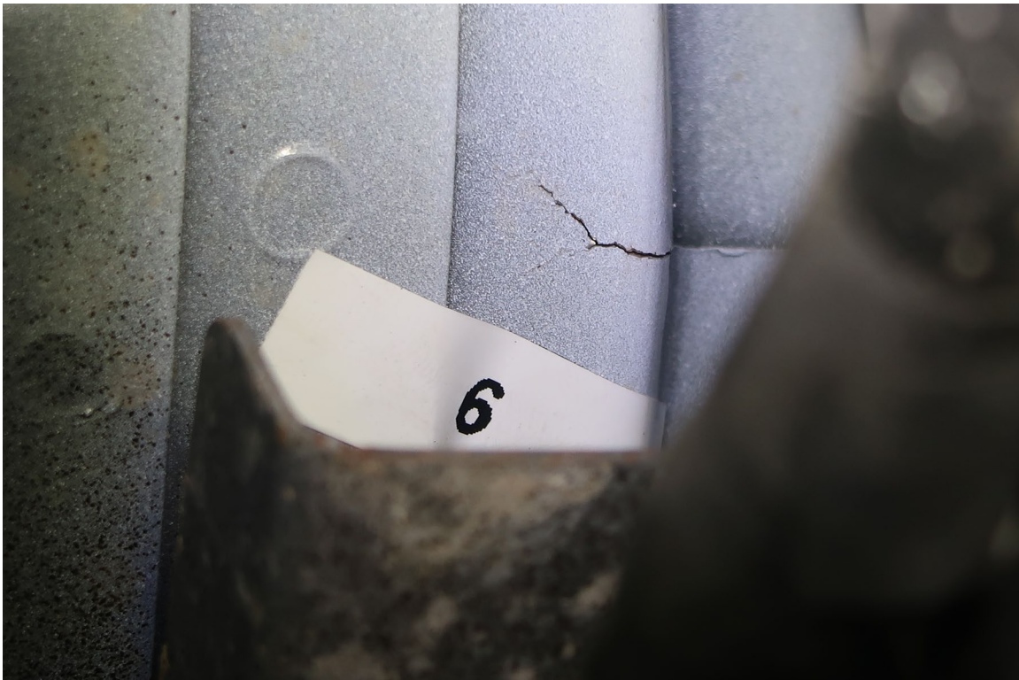
CRACK #6; CRACK IN THE CURBSIDE INNER FENDER STRUCTURE IN FRONT OF THE CURBSIDE ENTRANCE DOORSTEPS
