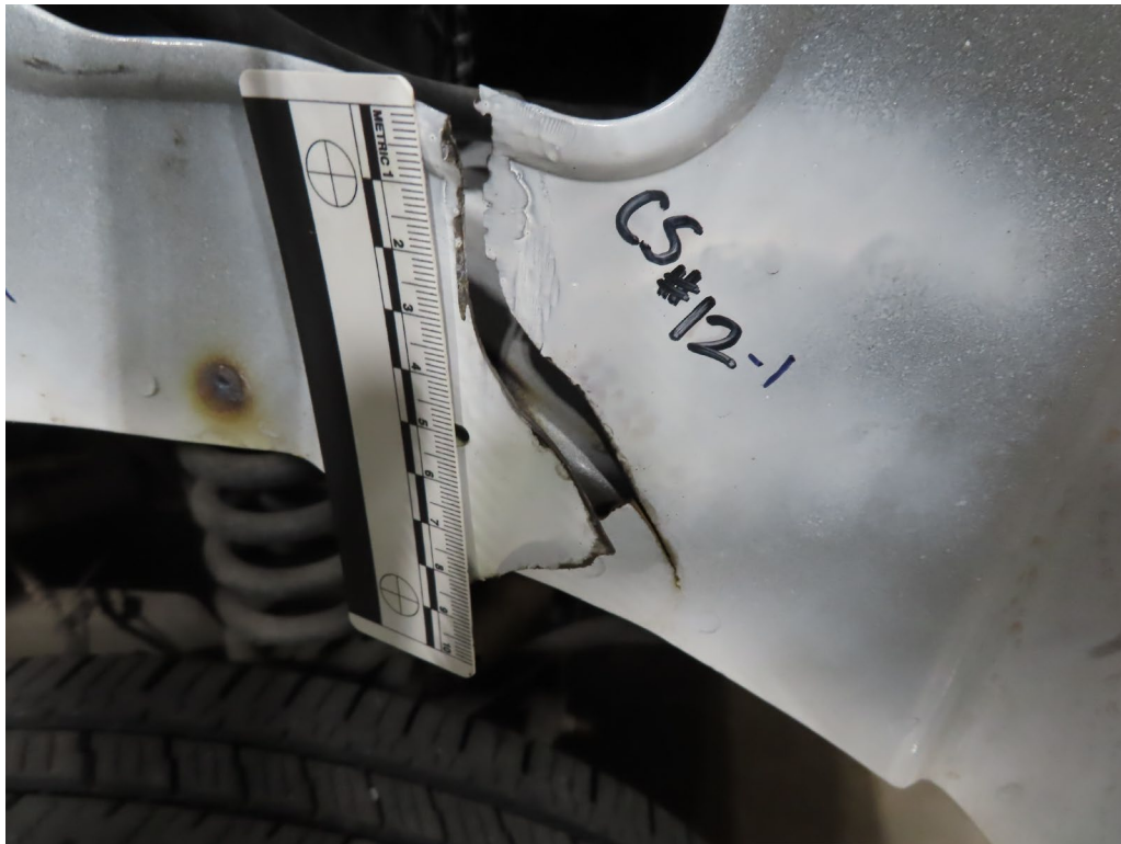
CRACK #12-1; WELDED REPAIR OF CRACK #12 ON THE CURBSIDE INNER FENDER HAS CRACKED
