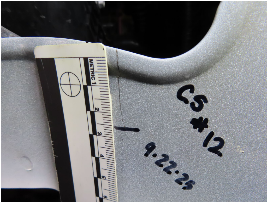
CRACK #12; CRACK ON THE CURBSIDE INNER FENDER
