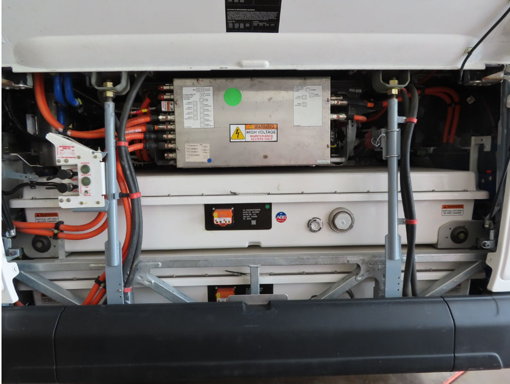
BATTERY PACKS IN REAR COMPARTMENT
